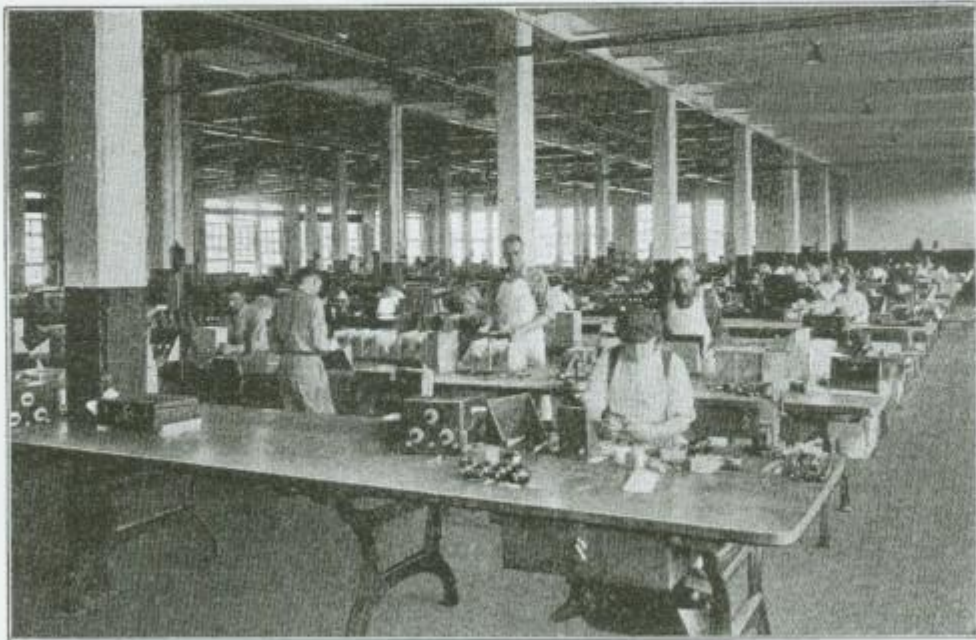
Section of Radio Assembling Room at Immense Plant of General Electric Company, Schenectady, N. Y.
