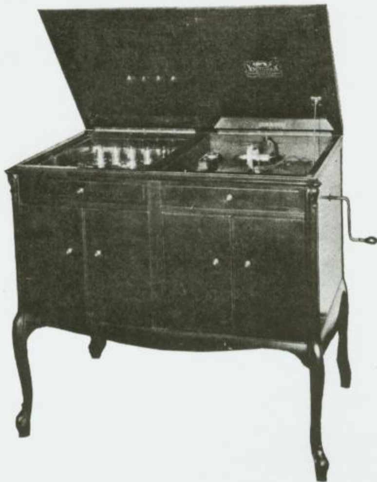
The Radiola IX as installed in Victor Victrola Model 220. The phonograph reproducer and the radio loud-speaker unit are easily interchangeable on the tone arm.
